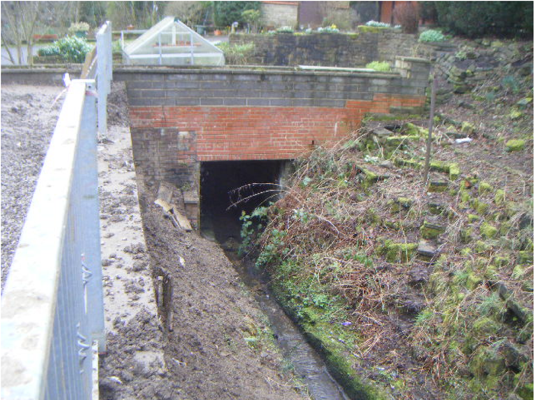
Photo showing downstream culvert
