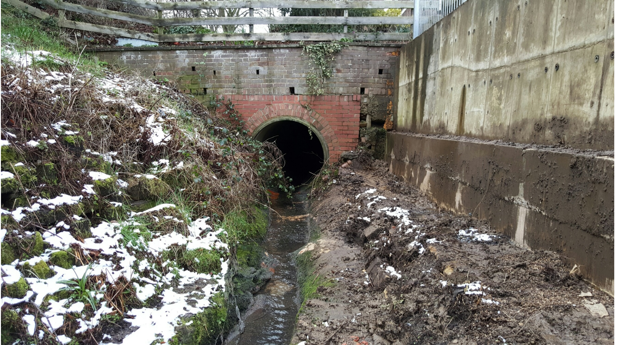
Photo showing upstream culvert
